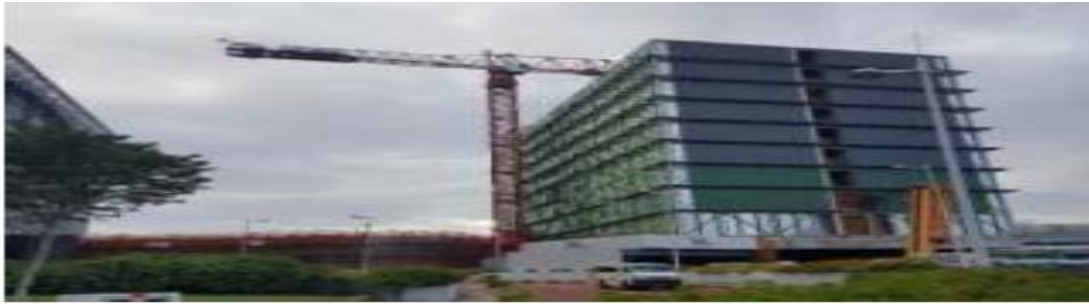
View of site from Terminal 2 during PPVC module installation
