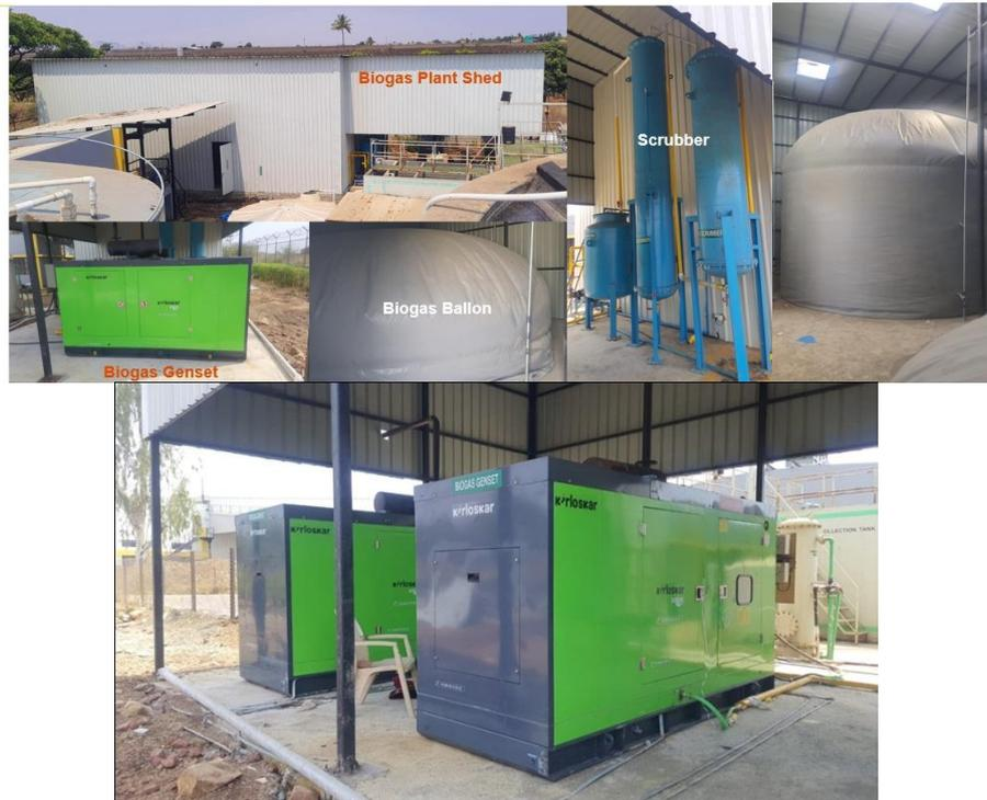
**Figure 3.** Images of the Bio-Gas Plant at Site, Sula Vineyards Limited
