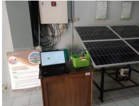
Figure 4. Solar Cell Installation
